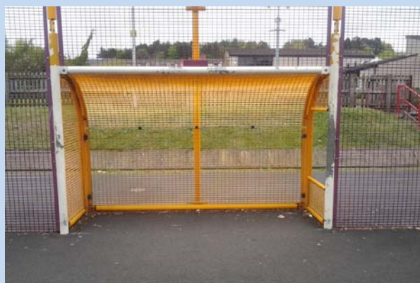
Paint damage on posts
